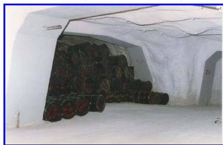
View of a Disposal Chamber in the Richard Repository
